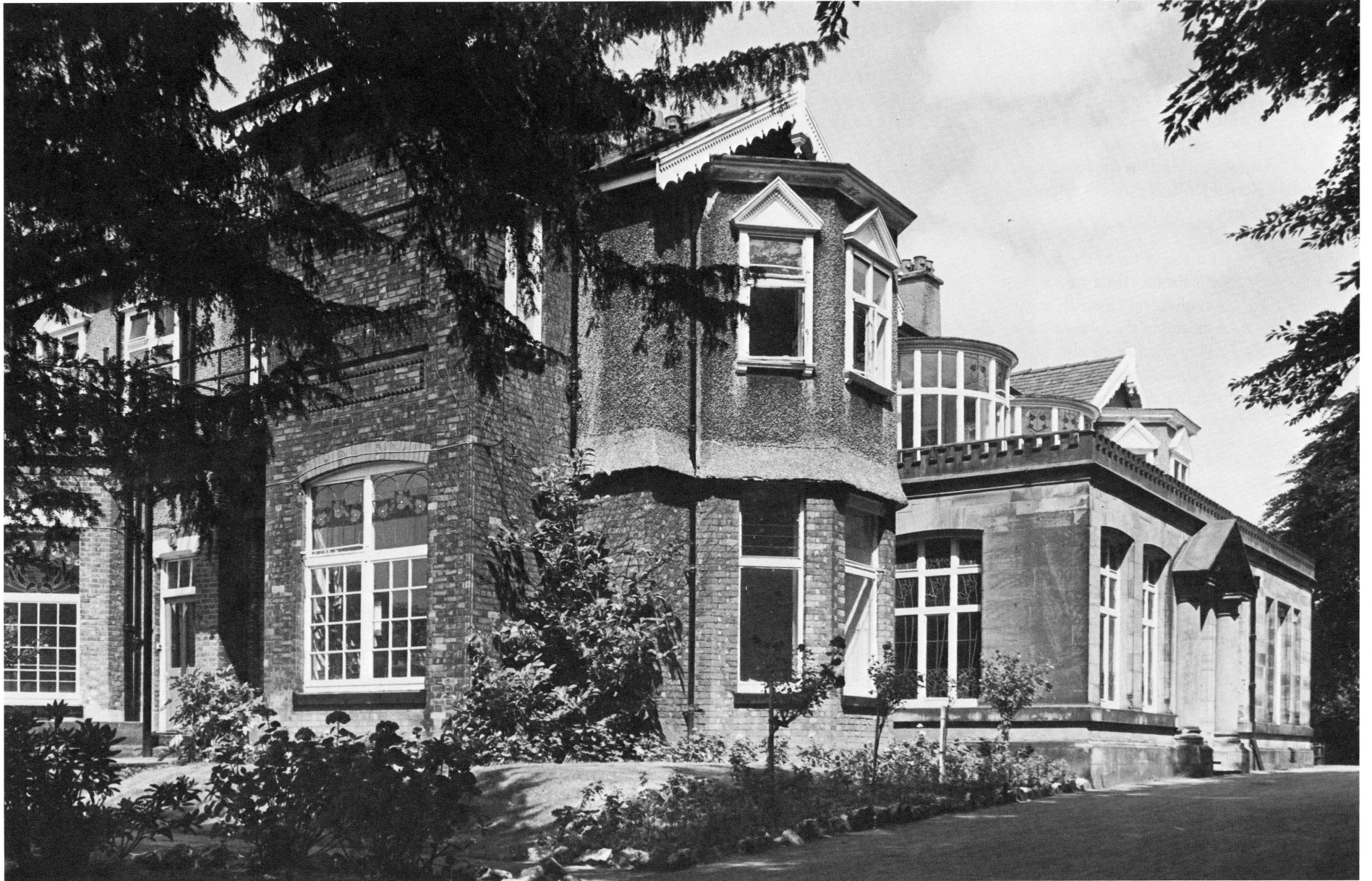
54 ROSE HILL Northenden near Manchester, exterior from the southwest.
